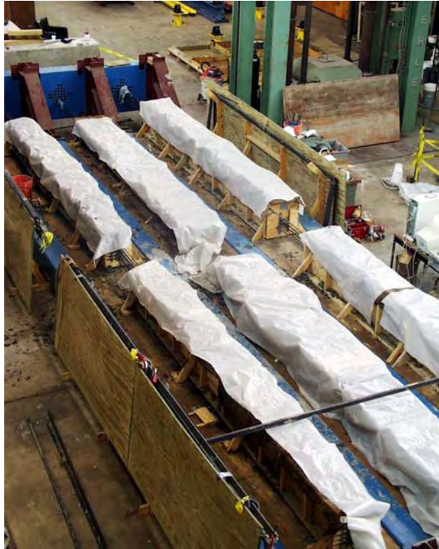
Figure B.3: Beams covered with wet burlap and plastic
