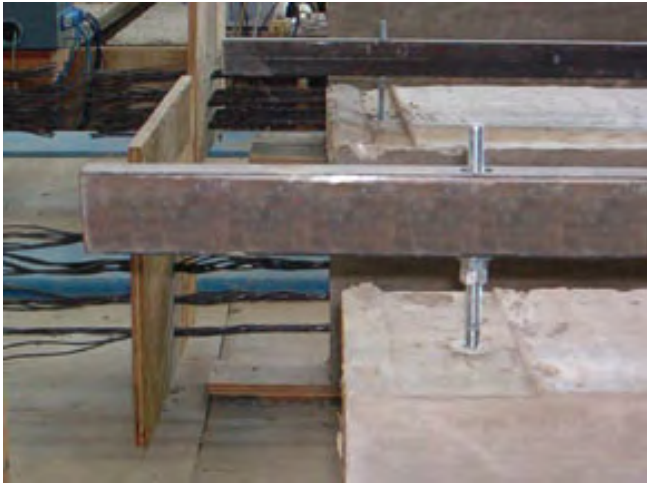
Figure 4-10: Support of frame for camber measurement
