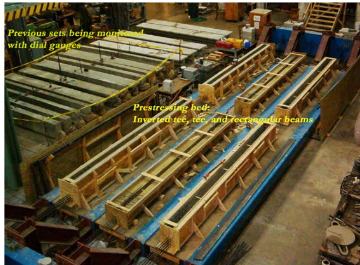
Figure B.1: Prestressing bed at Ferguson Laboratory
