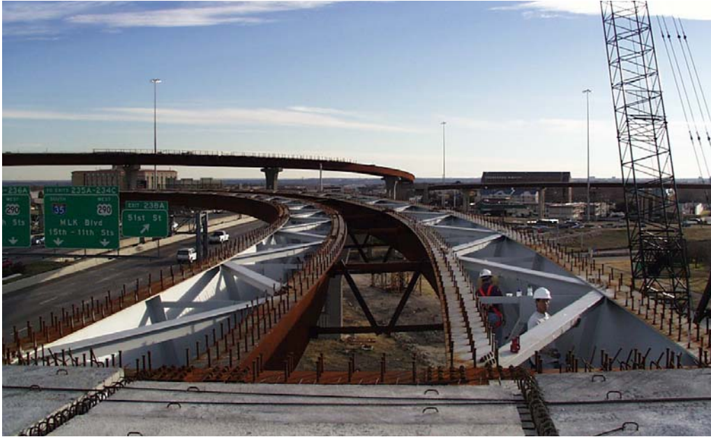
Figure 1.6 Bridge K during Construction (at 17K Looking South) (Cheplak, 2001)
