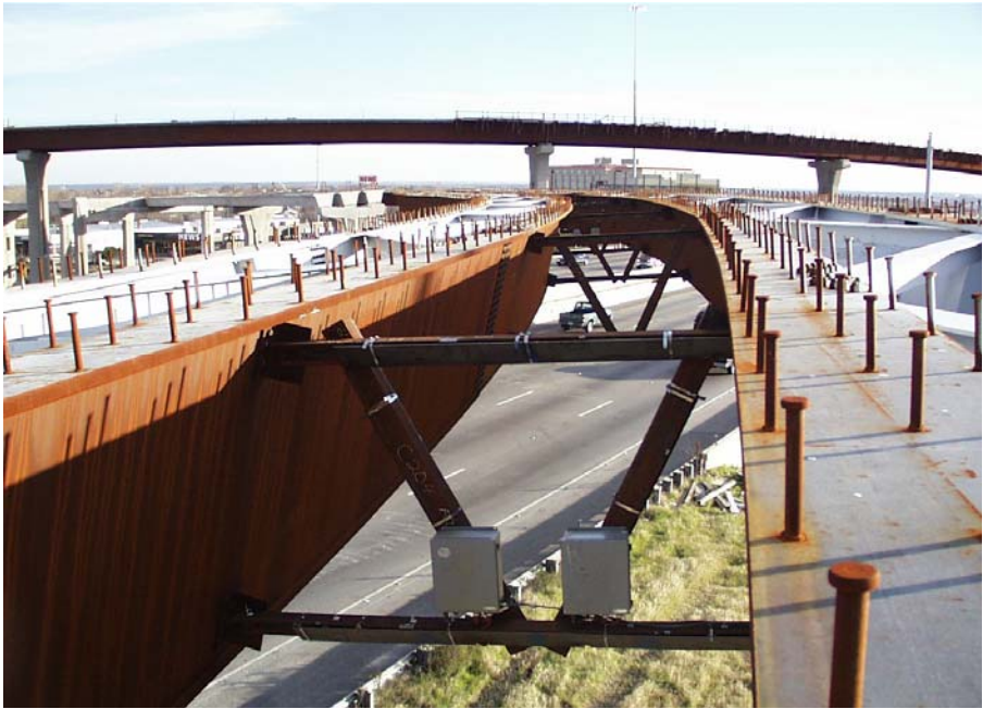
Figure 6.3 External Diaphragm #11 -- Looking South (Cheplak, 2001)
