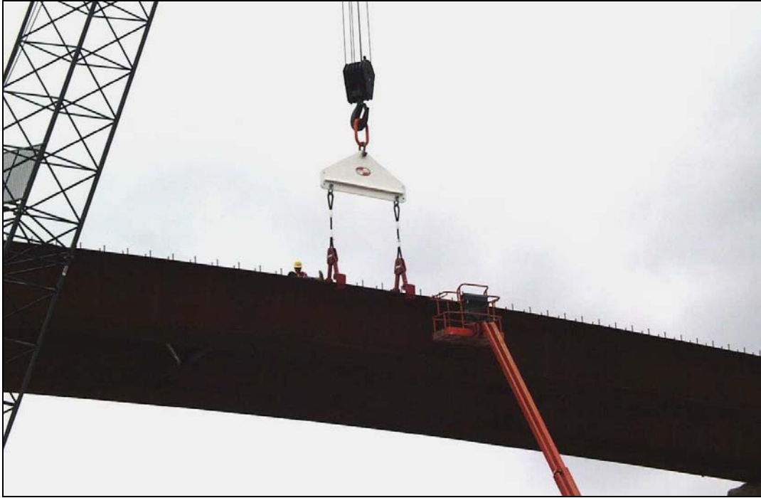
Figure 3.2 Crane Attachment
