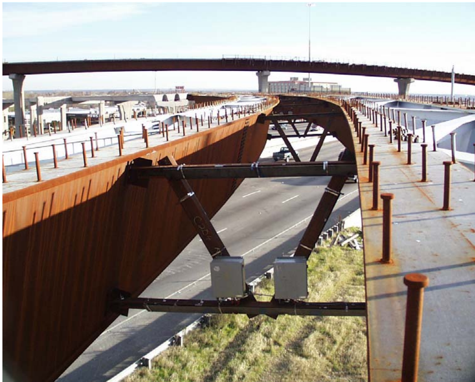
Figure 2.14 Intermediate External Diaphragm #11 -- Looking South
