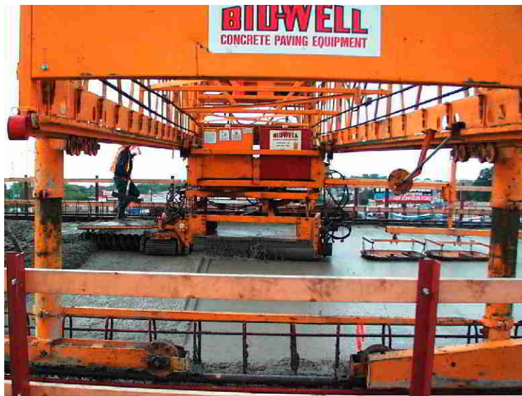
Figure 4.4 Concrete Screed
