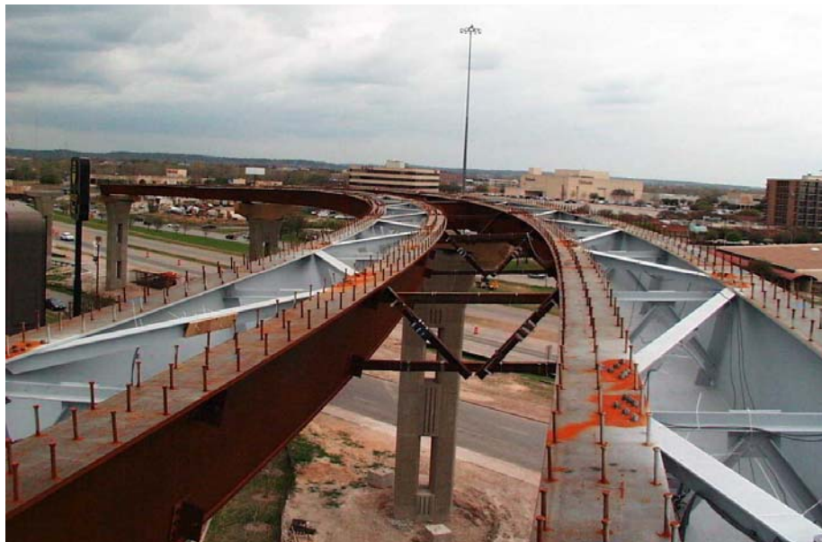
Figure 4.2 View of Z-Connect from Pier 16Z
