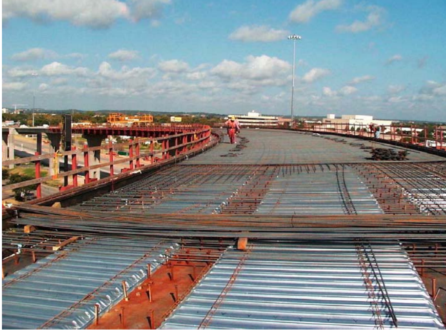
Figure 4.3 Deck Forms and Reinforcement Installation
