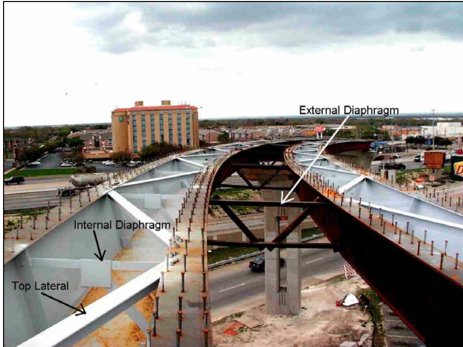
Figure 1.4 Picture of Z-Connect During Construction
