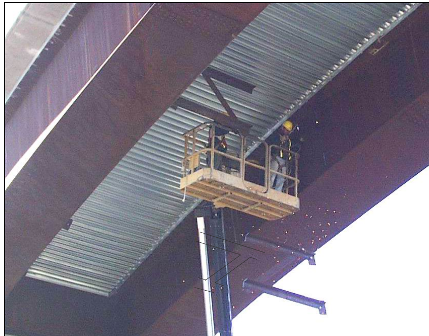
Figure 2.11 Flame Cut Removal of External Diaphragms
