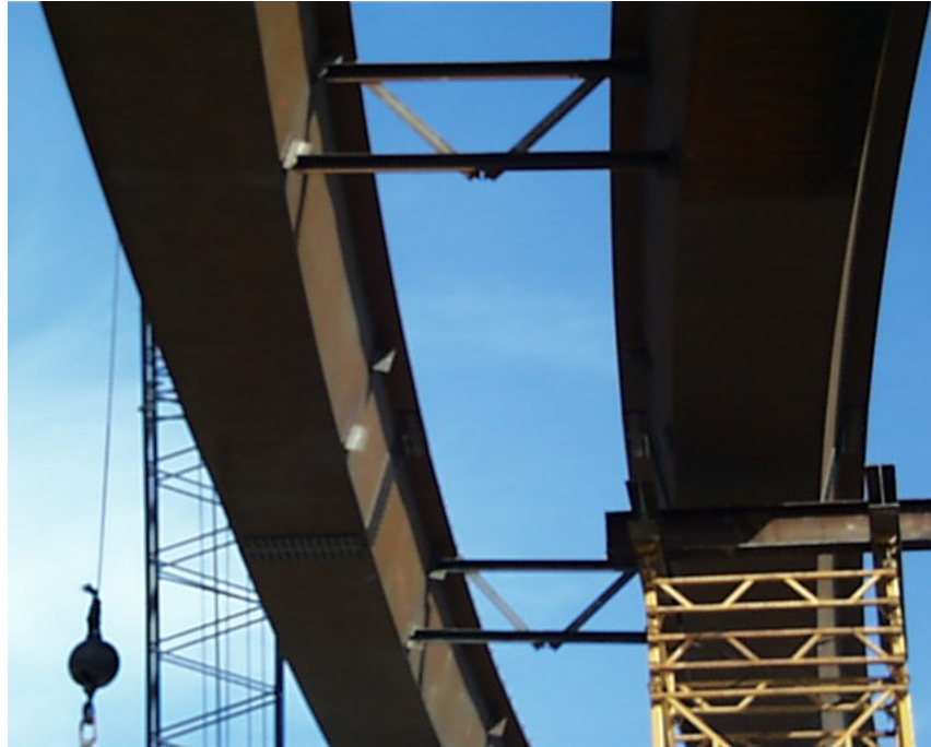
Figure 2.10 Installed External Diaphragms on Z-Connect
