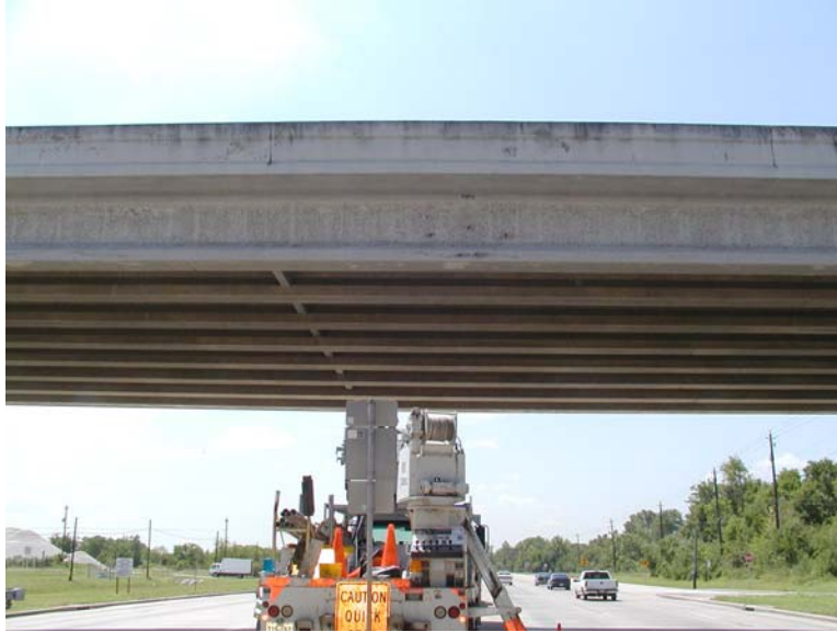
Figure 7.25: Overall view of Points 3-5, Beltway 8 (facing south) (6/22/01)
