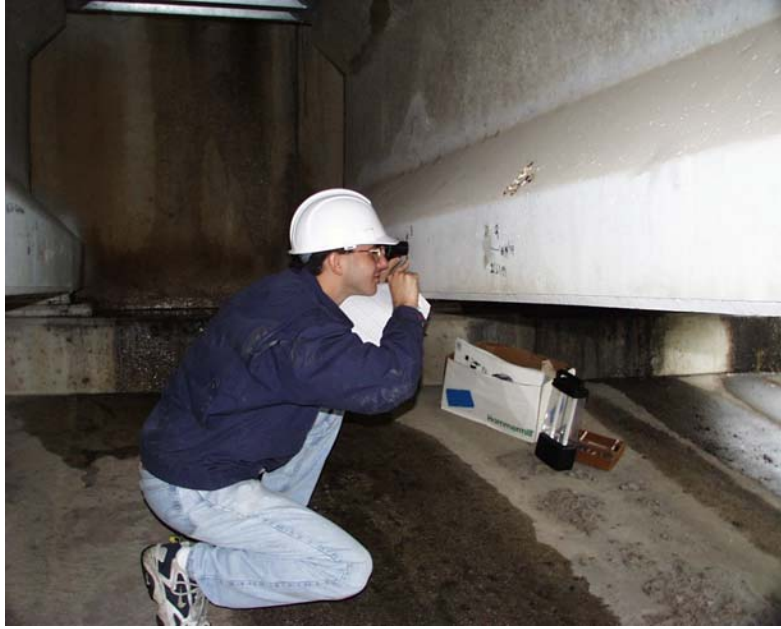
Figure 6.11: Measuring crack widths with optical scope
