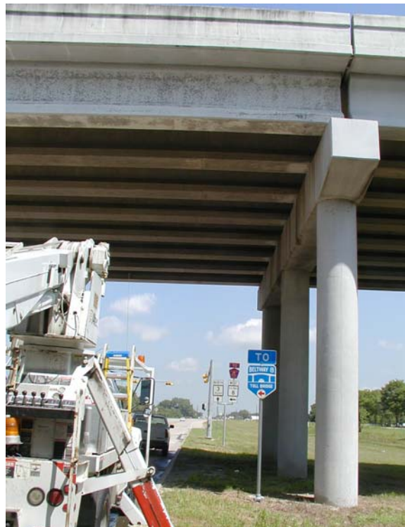
Figure 7.29: Overall view of Point 7, Beltway 8 structure (facing north) (6/22/01)
