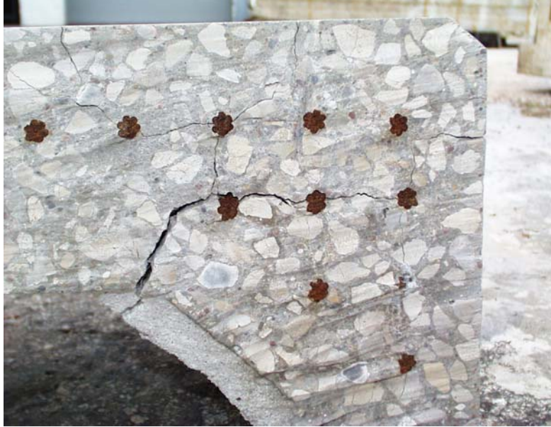
Figure 3.15: Large cracks in back face of Slice BG2N
