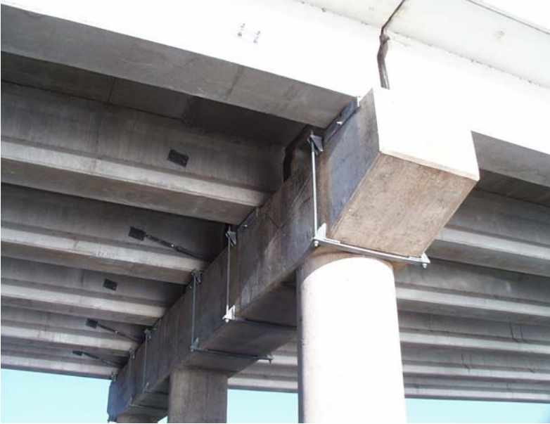
Figure 7.36: Overall view of Bent 5 (facing north)
