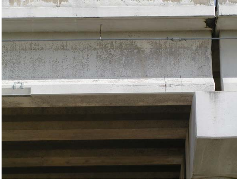
Figure 7.26: Overall view of Point 1, Beltway 8 structure (facing north) (6/22/01)
