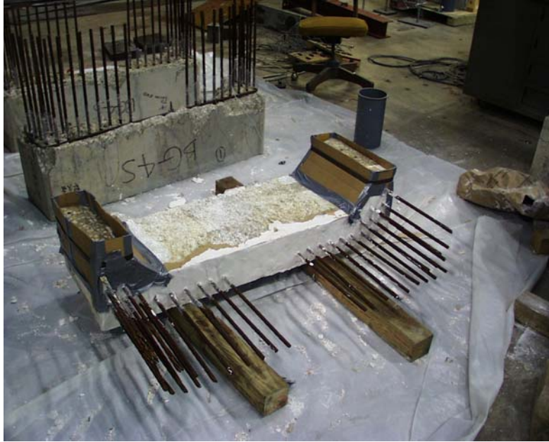
Figure 3.25: Formwork for web sections
