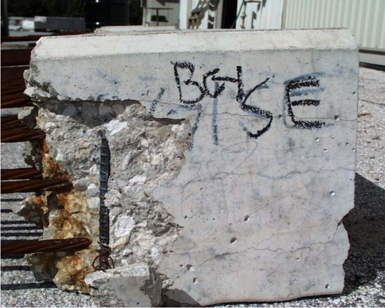
Figure 3.12: Cracking on left face of Slice BG1S
