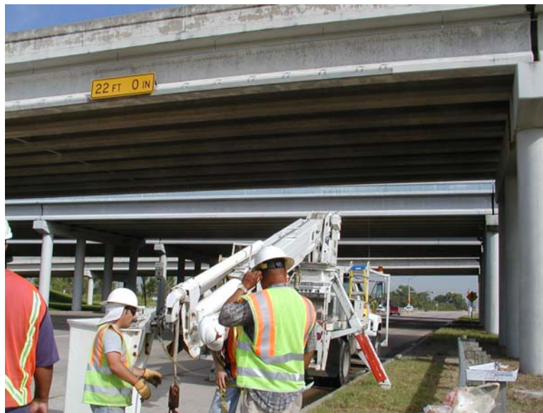
Figure 6.7: Beltway 8 over State Highway 3, Houston, Texas (facing north)
