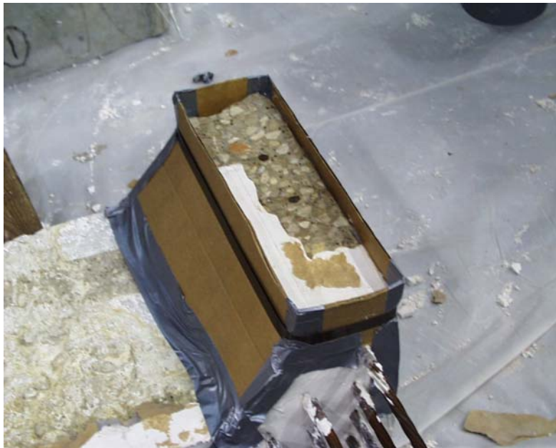
Figure 3.26: Cardboard formwork for top of web
