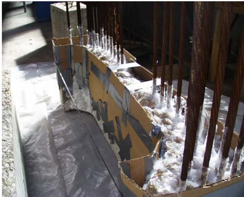
Figure 3.24: Cardboard formwork used for front face
