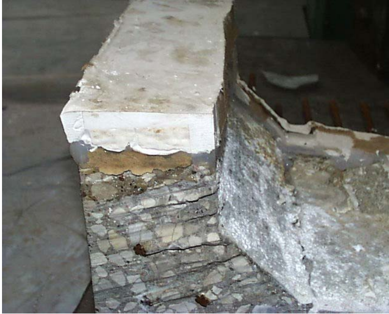
Figure 3.27 Level Hydrostone bearing surface on top of web section
