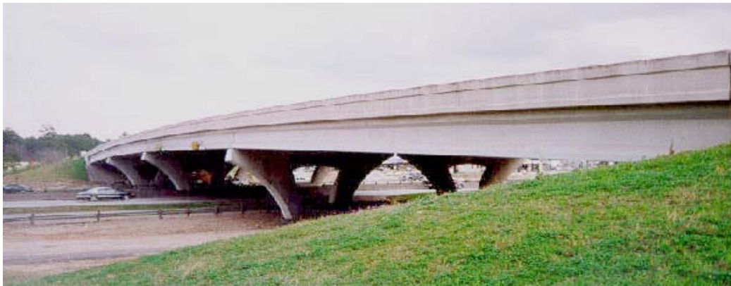
Figure 6.5: Robinson Road over I-45 in The Woodlands, Texas
