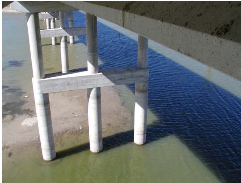
Figure 7.38: Overall view of Bent 9 (facing west)
