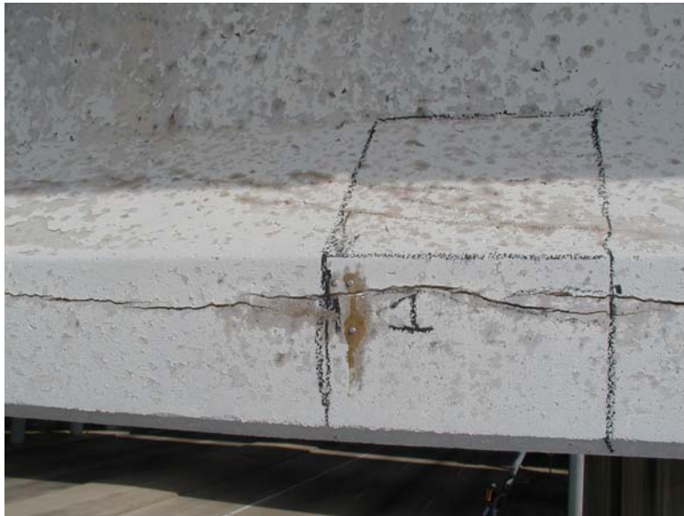
Figure 7.27: Close-up view of Point 1, Beltway 8 structure (6/22/01)
