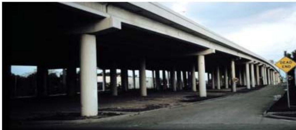
Figure 6.1: I-10 over AT & SF RR in Beaumont, Texas (facing east)
