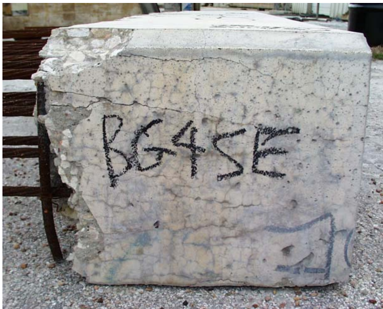
Figure 3.18: Cracking on left face of Slice BG4S1
