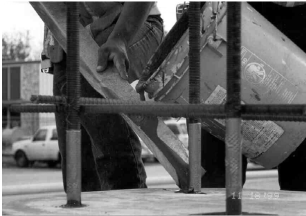
a. Gravity-flow Grouting
