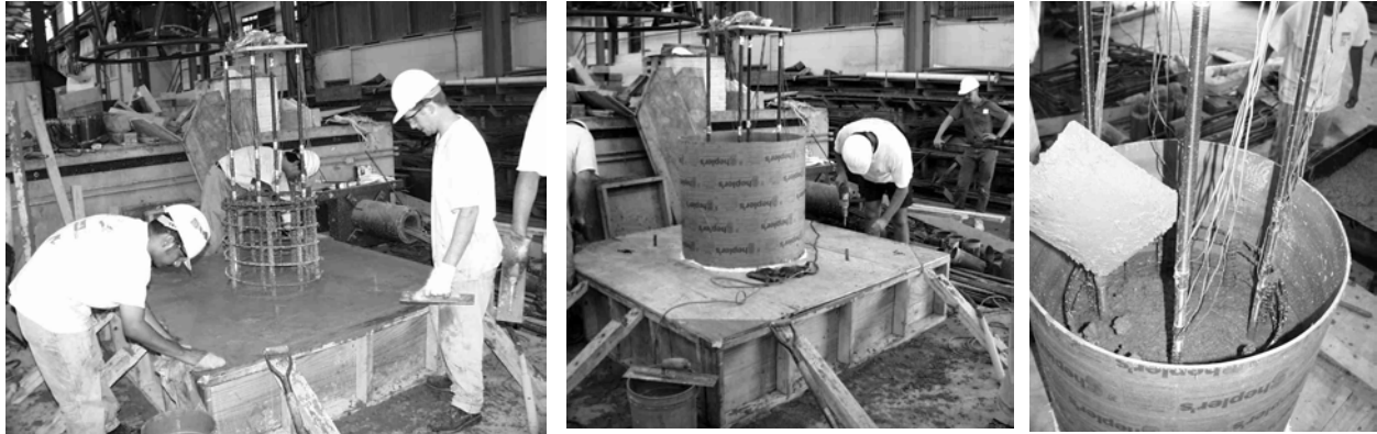
a. Casting Footing
