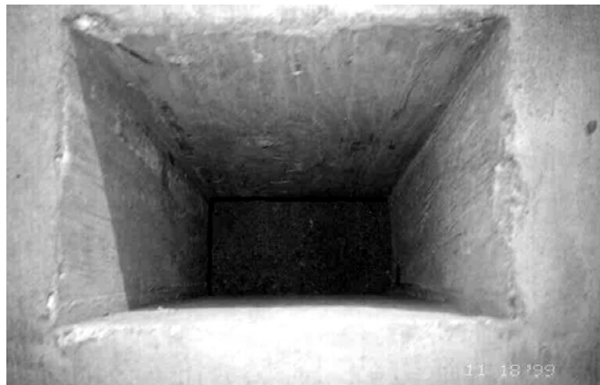
Figure 5.14 Single-line Grout Pocket after Form Removal
