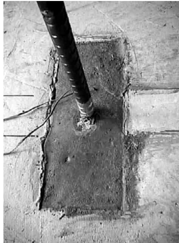
Figure 3.23 Single-Line Grout Pocket after Curing
