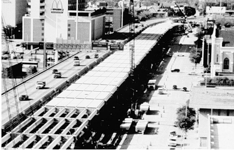
Figure 1.3 View of Pierce Street Elevated Project During Construction
