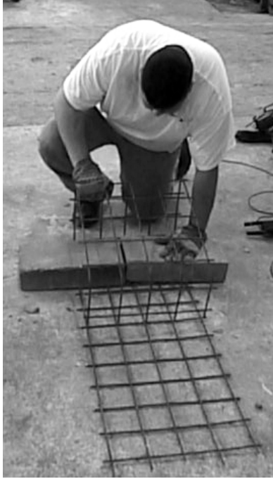
Figure 3.13 Preparation of Welded Wire Fabric Confinement
