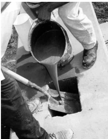
a. Placement with Bucket
