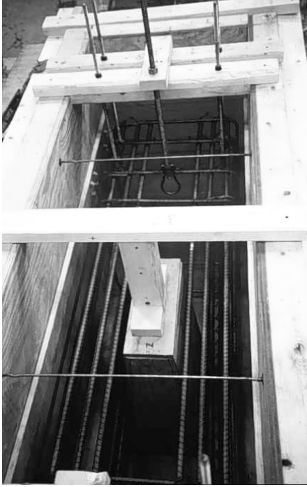
Figure 3.7 Single-Line Rebar Cage
