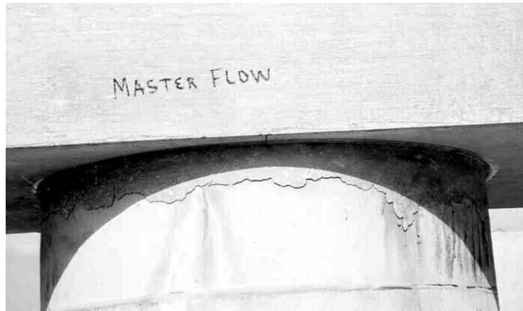
Figure 5.22 Bedding after Tremie-tube Grouting
