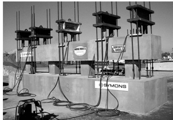
b. Pile Bent Test Setup
