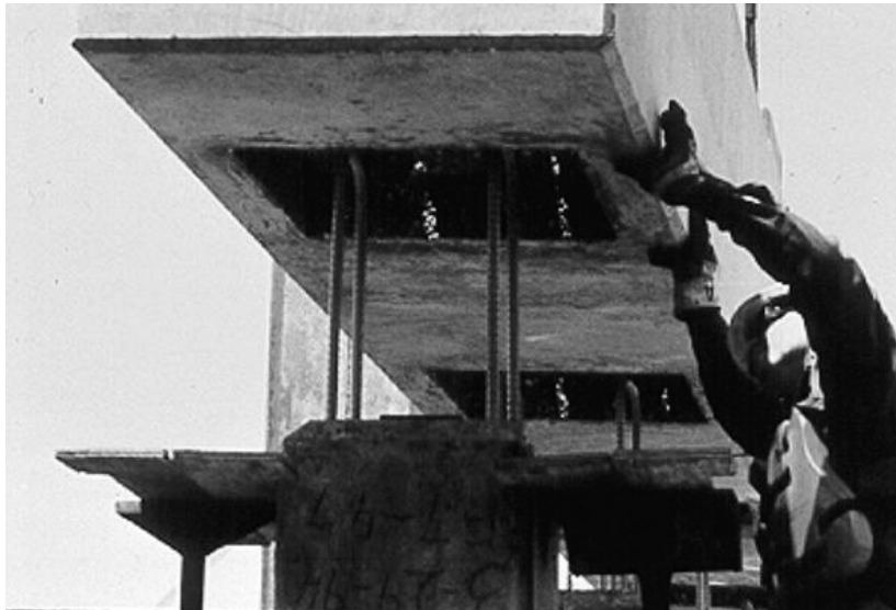
Figure 1.9 Lowering of Precast Cap over Dowels
