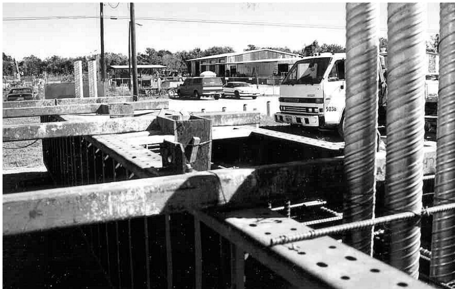
Figure 5.7 Pile Cap Formwork
