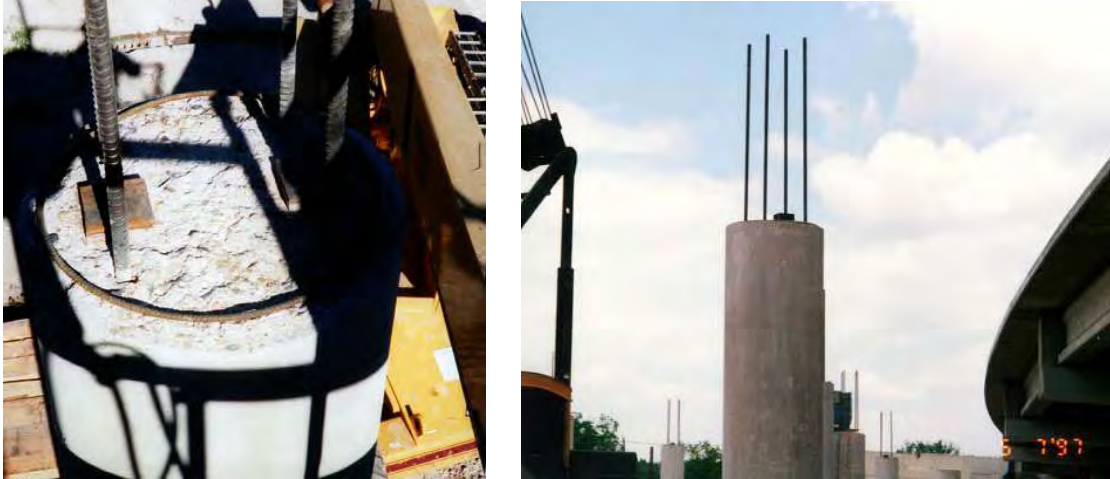
Figure 2.5 Shims at top of Column in Pierce Street Elevated Project
