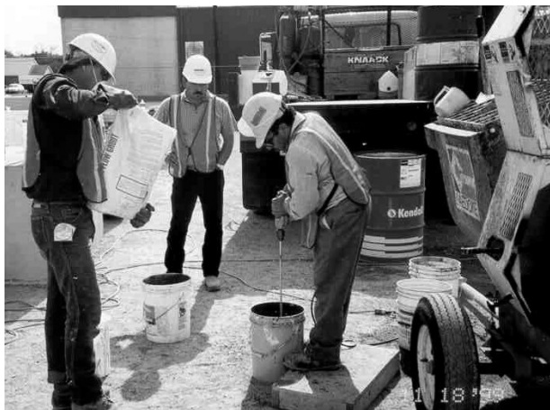
a. Grout Mixing
