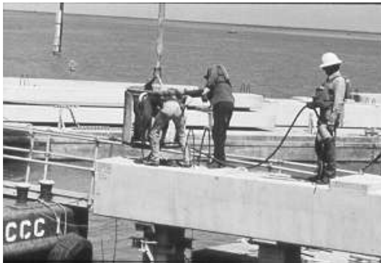
Figure 1.11 Workers Casting Concrete into Grout Pocket
