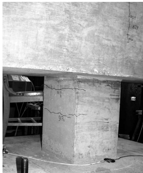
Figure 4.43 PSL3 Pile Cracks (NE) at Factored-Level Load
