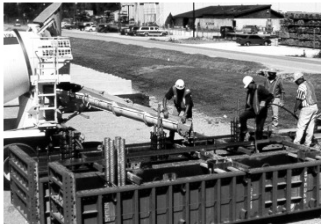
Figure 5.13 Casting of Bent Caps
