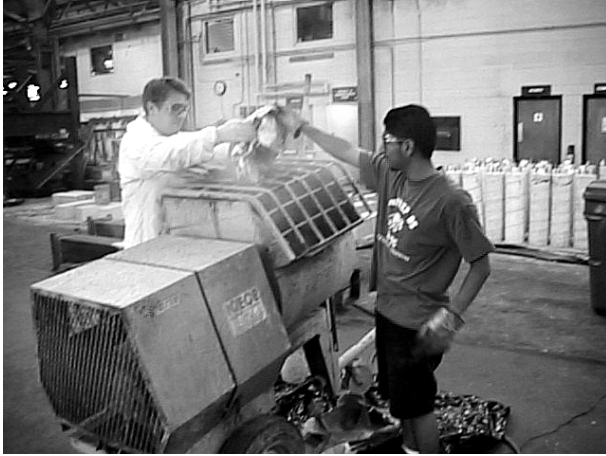
Figure 3.21 Grout Mixing
