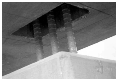
b. Single Line Grout Pocket
