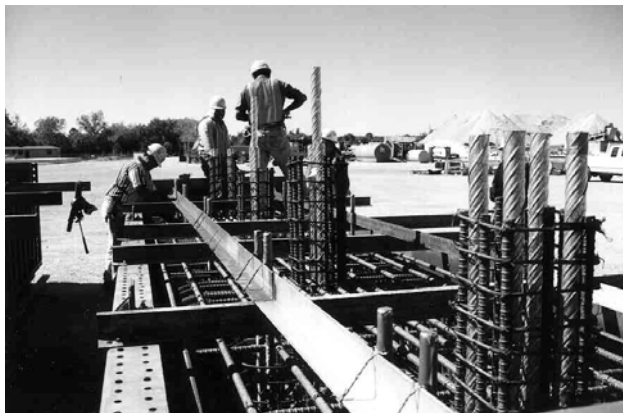
a. Pile Bent Construction
