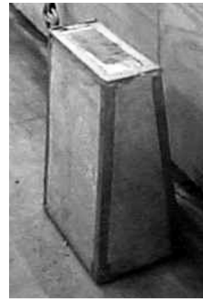
Figure 3.10 Single-Line Grout Pocket Insert
