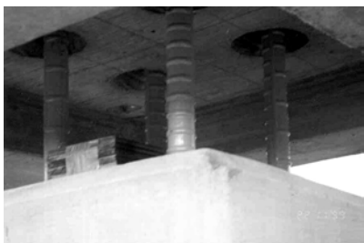
a. Vertical Duct
