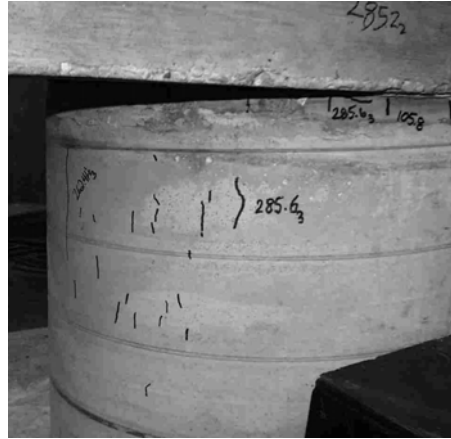
b. Cracks on Compression Side
