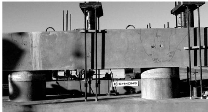
Figure 5.46 Flexural Cracks for CB2
