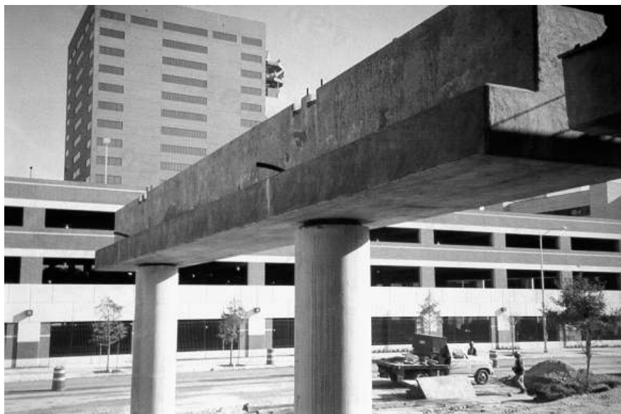
Figure 1.1 Precast Bent Cap on Pierce Street Elevated Project
