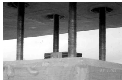
c. Bolted Connection
