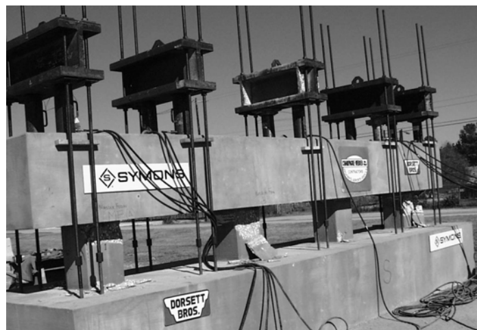
Figure 5.42 Crushing and Spalling at Pile Tops in PB3—Front View
