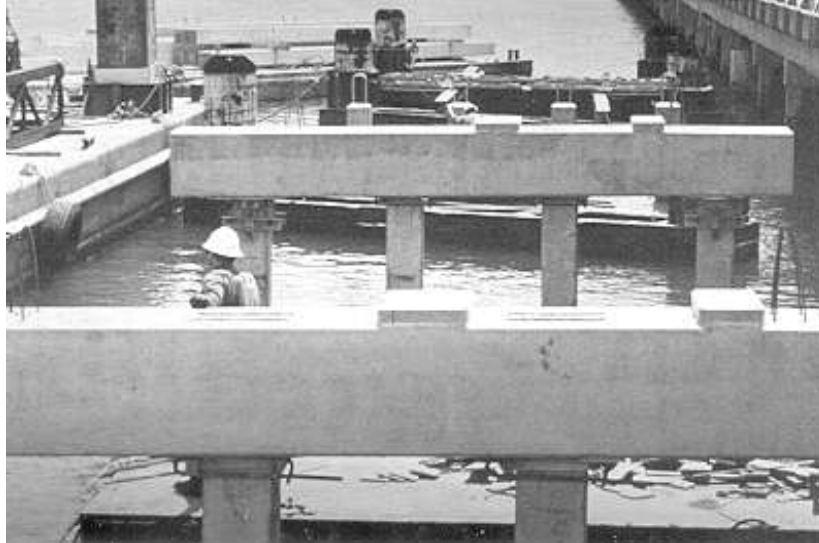
Figure 1.2 Precast Bent Caps on Red Fish Bay Project
