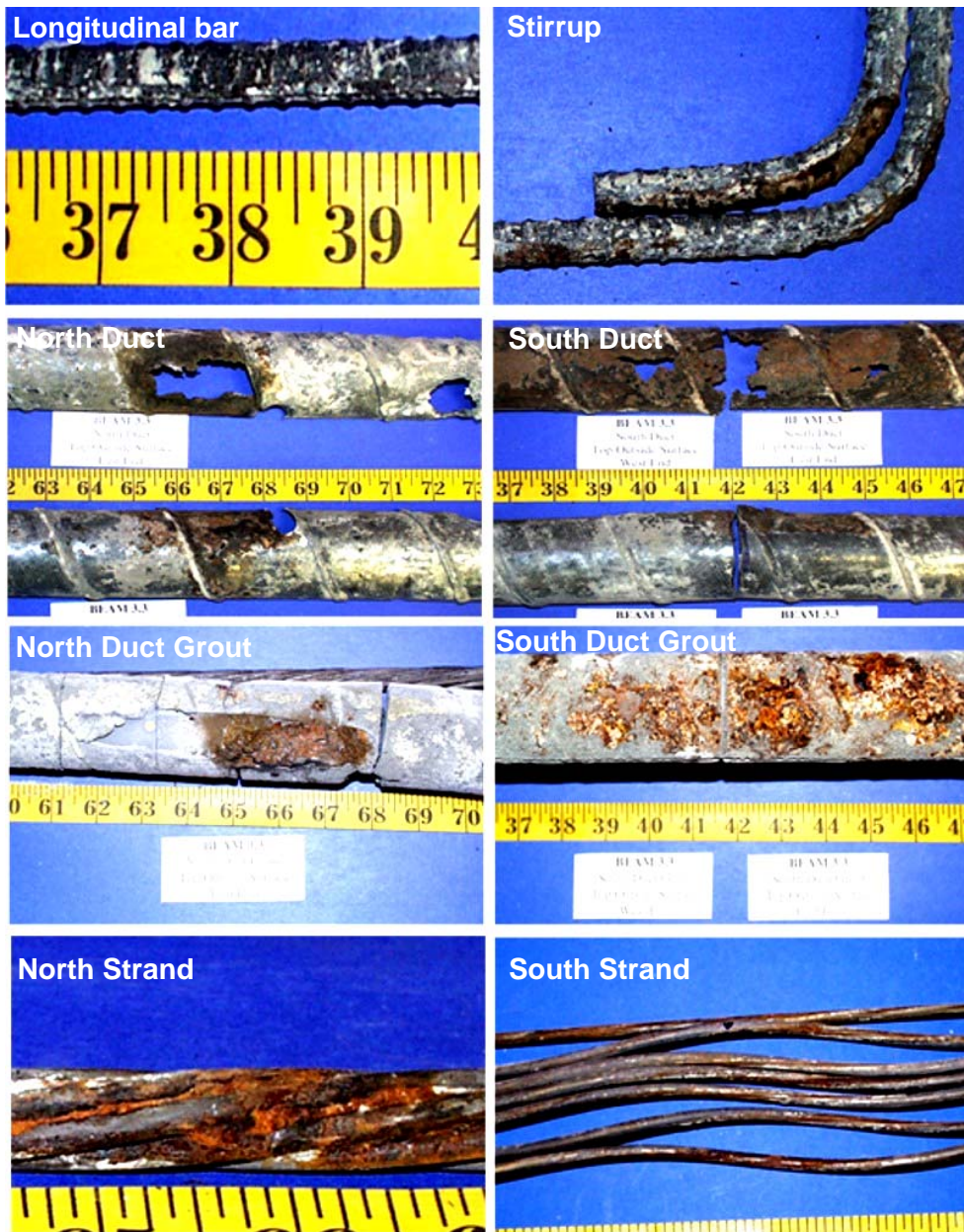
Figure 5.34 Specimen 3.3 – Reinforcing Elements 6,7
