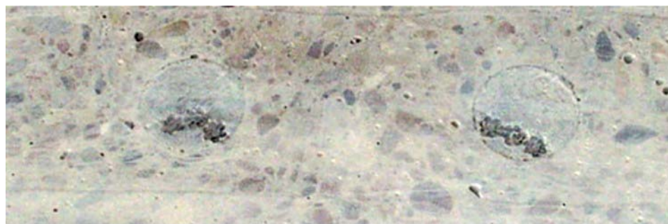
Figure 5.28 Specimen 3.2 – Grouted Duct 6,7
