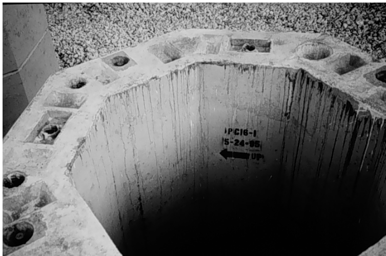
Figure 1.5 - Precast Bridge Pier Segment Close Up
