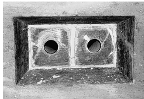
completed end pocket
