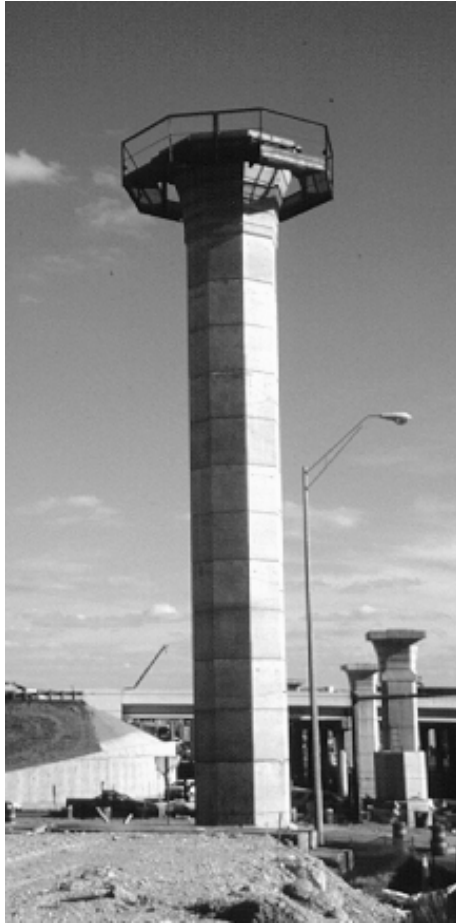
Figure 1.4 - Post-Tensioned Precast Segmental Bridge Pier
