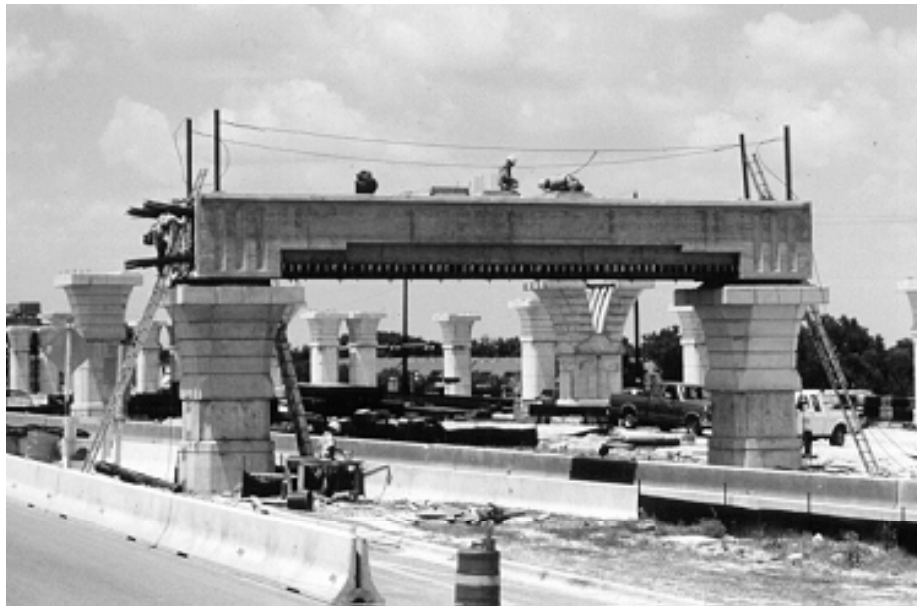
Figure 1.7 - Post-Tensioned Straddle Bent
