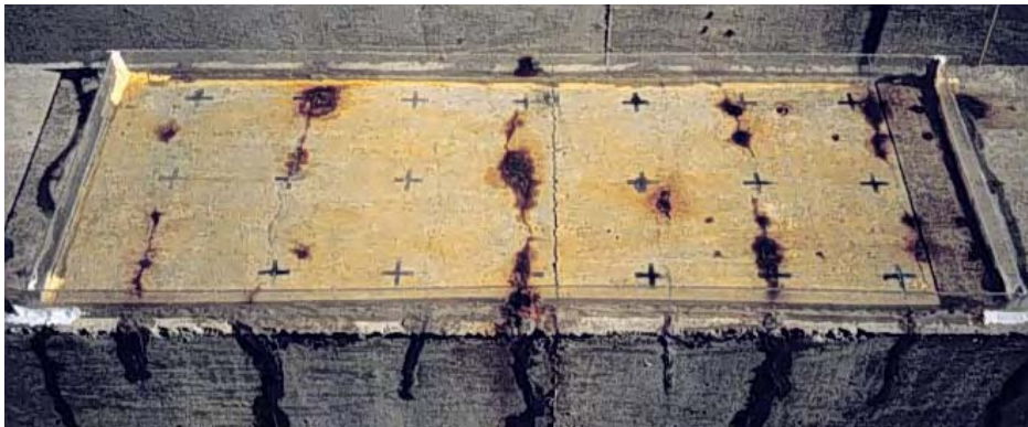
Figure 2.96 - Staining on Specimen 1.3
