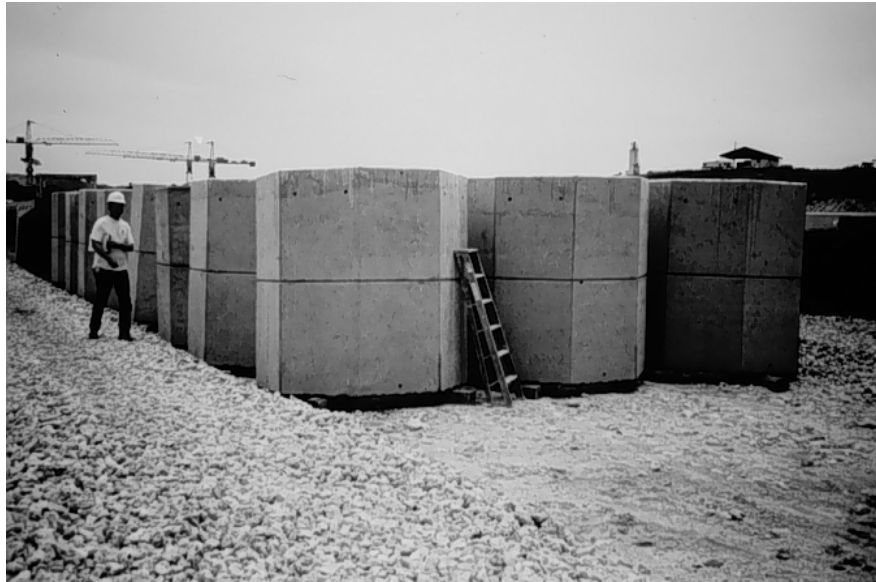
Figure 1.6 - Precast Bridge Pier Segments
