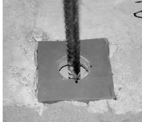
Gasket Around Post-Tensioning Bar
