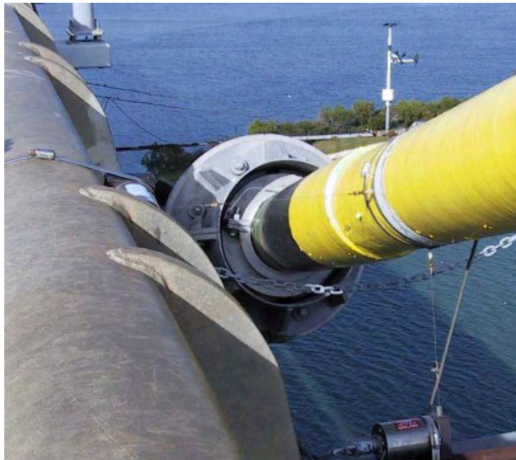
Figure 6.22 Freyssinet damper installed on stay AS24
