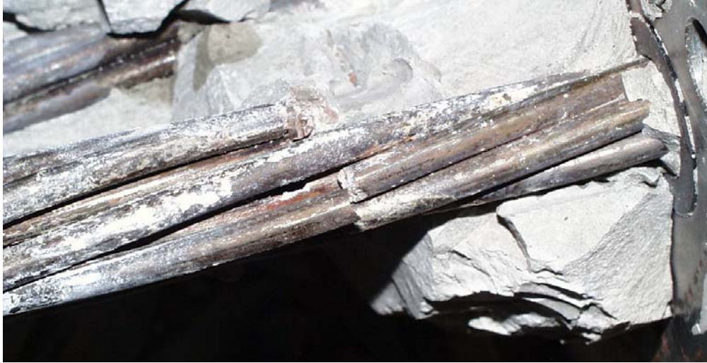
Figure D.65 Wire Breaks in Strand 1 near Tower End – Specimen 6
