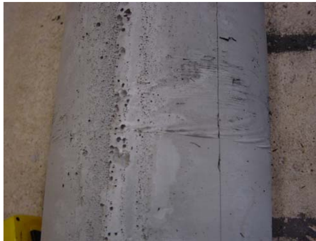
Figure D.37 Distributed Air Voids at Tower End of Specimen 3
