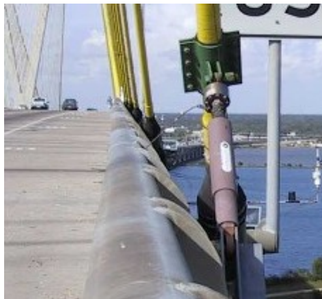
Figure 5.1 Hydraulic Damper Installed on the Fred Hartman Bridge
