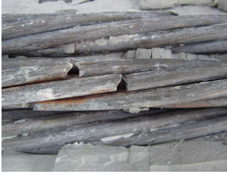
Figure D.17 Wire Breaks in Strand 1 near Midspan of Specimen 1
