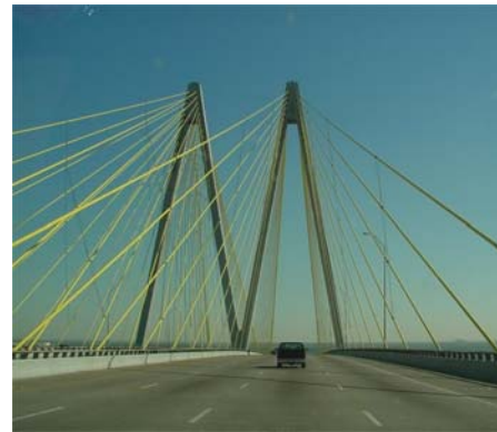
Figure 1.2 Fred Hartman Bridge
