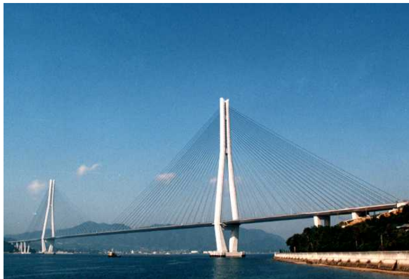
Figure 1.3 Tatara Bridge, Japan
