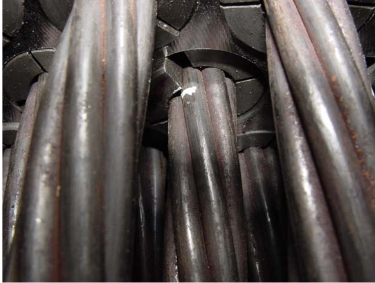
Figure B.34 Unequally Seated Wedges at the Deck End of Specimen 1
