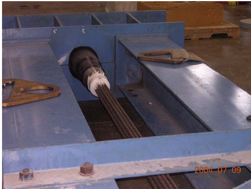
Figure B.31 PVC Cap in Position Adjacent to Tension Ring in Hybrid Specimen
