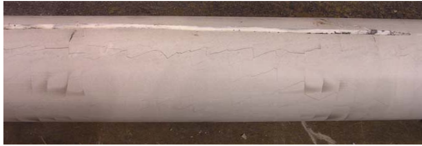
Figure D.136 Condition of Grout under Load Point – Specimen 11
