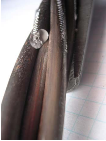
Figure D.100 Wire Break in Strand 9 at Deck End of Specimen 8
