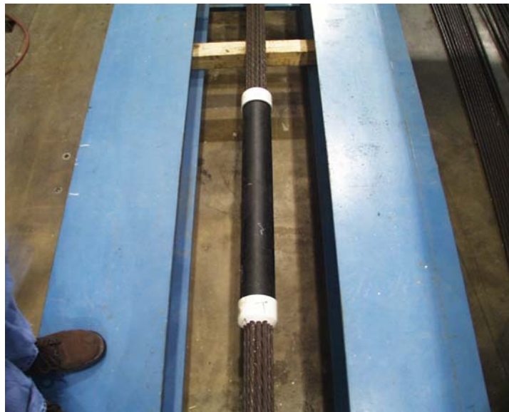
Figure B.28 PE Pipe and PVC End Caps used at Midspan of UngROUTED Specimens
