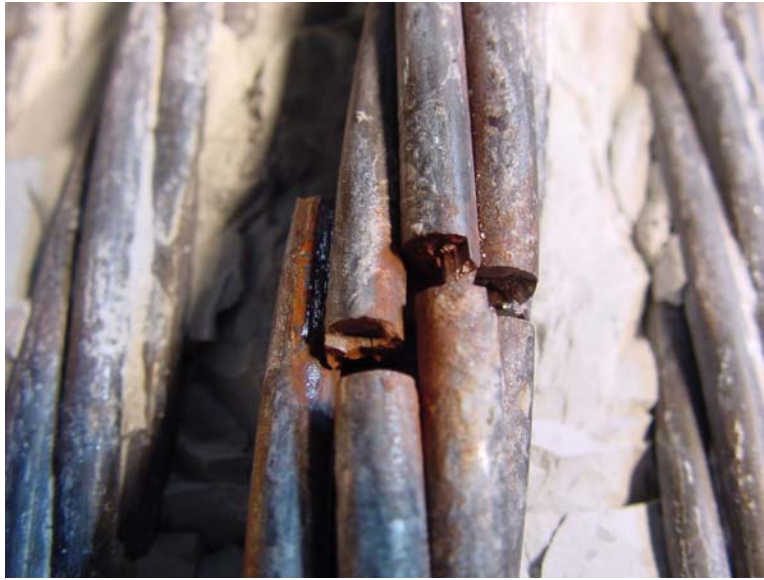
Figure D.15 Wire Breaks in Strand 19 near Tower End of Specimen 1
