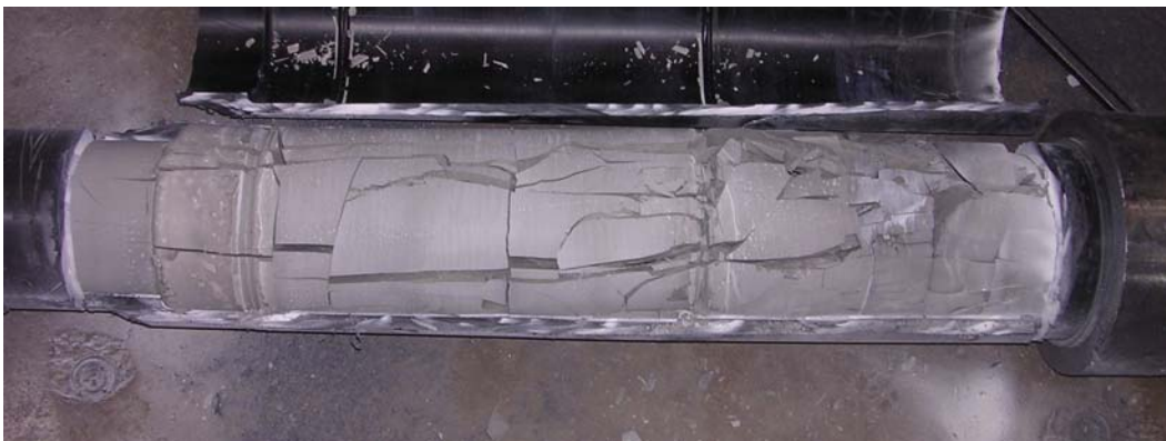
Figure D.122 Condition of Grout at Deck End Immediately after Removing PE Pipe – Specimen 10
