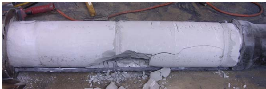
Figure D.135 Condition of Grout near Deck End – Specimen 11
