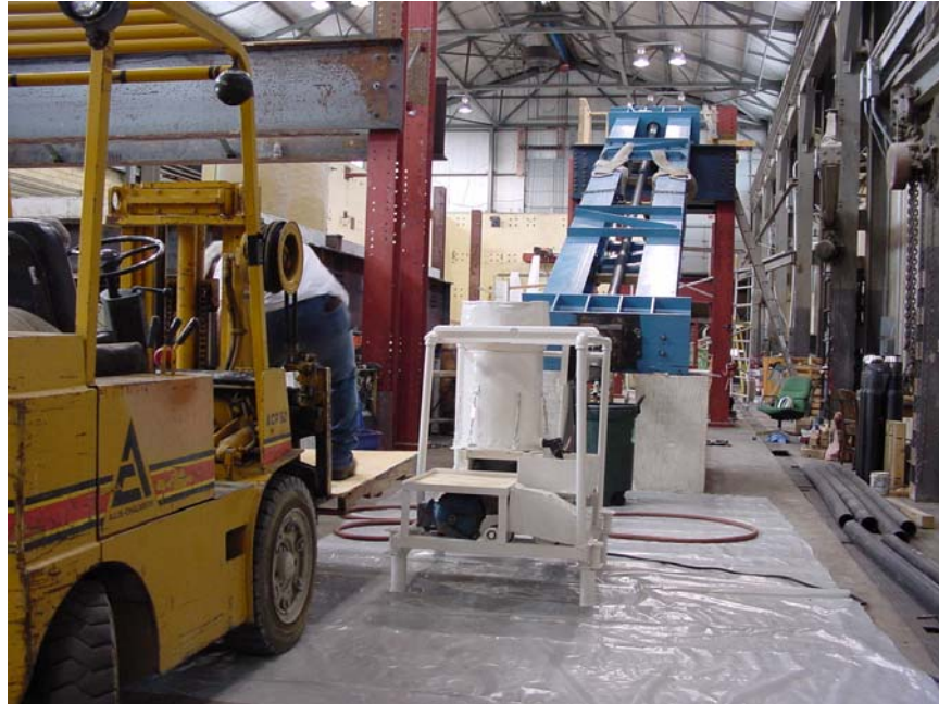
Figure 2.4 Position of Cable-Stay Specimen during Grouting
