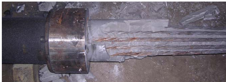
Figure D.150 Corrosion on Surface of Strand near Deck End – Specimen 12
