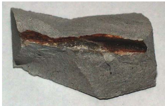
Figure D.62 Corrosion Product on Grout from Tower End of Specimen 6
