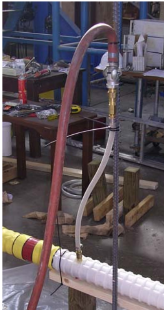
(a) Grout Hose from Pump
