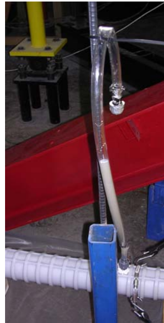
(b) Vent Hose after Completion of Grouting
