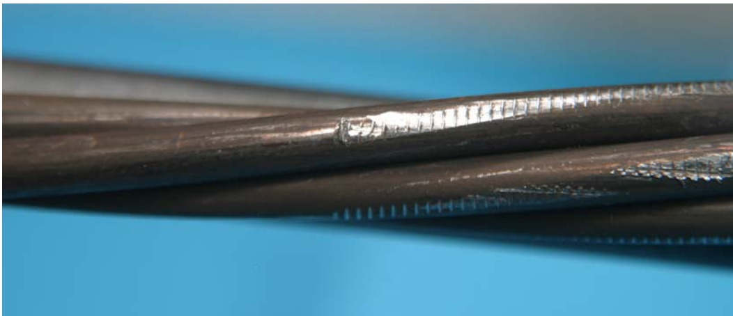
Figure D.97 Scraping of Strand Due to Stressing at Tower End – Specimen 8
