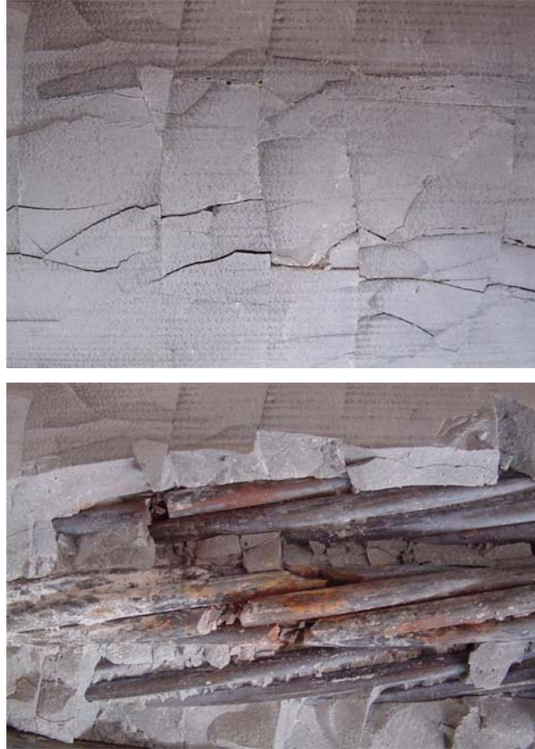
Figure 3.11 Longitudinal Cracks in Grout, Corrosion of Strand, and Wire Breaks near Midspan of Specimen 1
