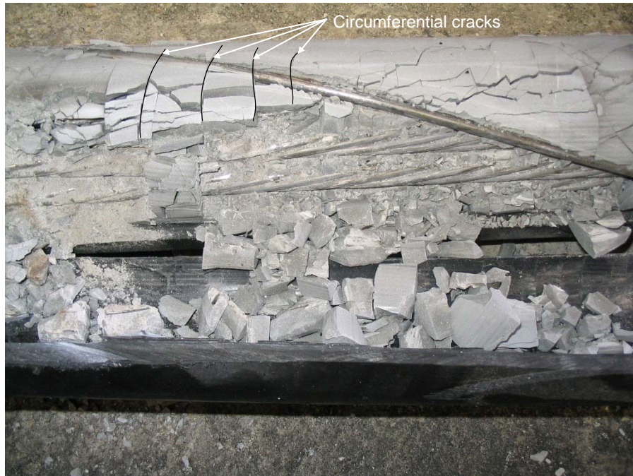
Figure D.75 Condition of Grout under Load Point – Specimen 7
