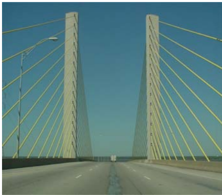
Figure 1.1 Veterans Memorial Bridge
