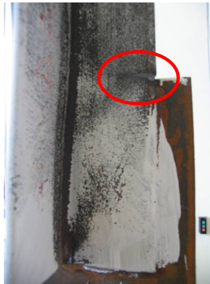
Figure 33. Typical Static Failure of Angle
