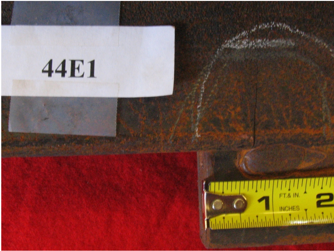
Figure 39. 44E Angle Failure Close-Up
