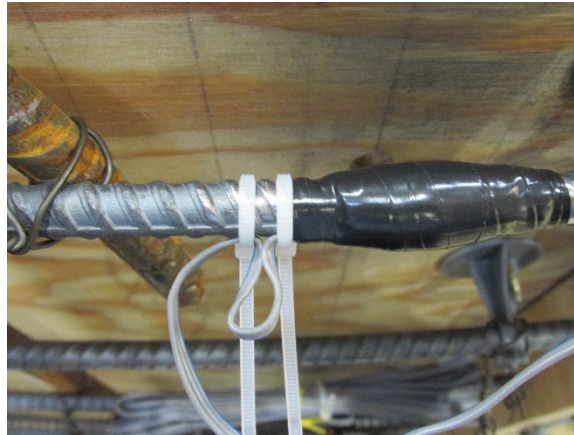
Figure 17 – Zip ties applied to wire for protection
