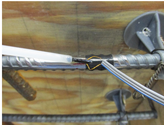
Figure 11 – Application of M-Coat A to exposed lead wires
