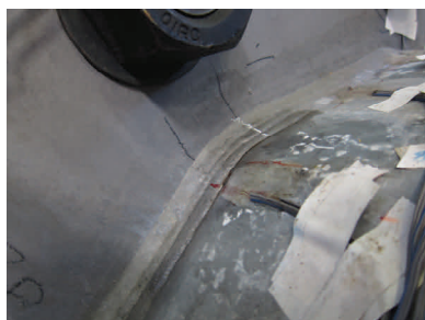
Figure 1: Fatigue cracks begin to propagate near the extreme tension fiber of specimen
