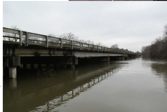
Figure 2: Bridge to be strengthened (with record high river levels flowing beneath)
