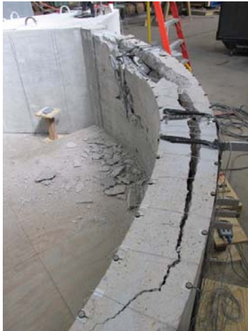
Figure 1: Cracked specimen 1 after the test
