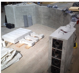
Pilot test specimen after formwork removal
