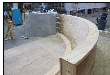
Outside wall formwork
