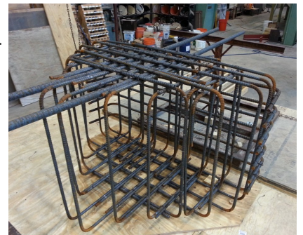
Steel cage for end block of first specimen
