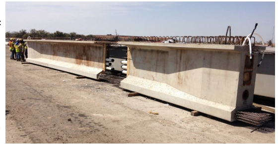
Precast segments for the upcoming splice region test
