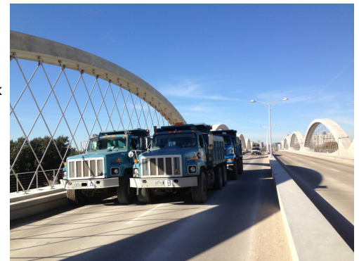
A truck load test being performed on the arch bridge
