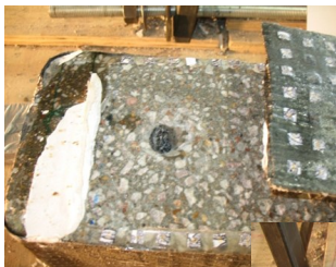
Above: Anchor failure mode
