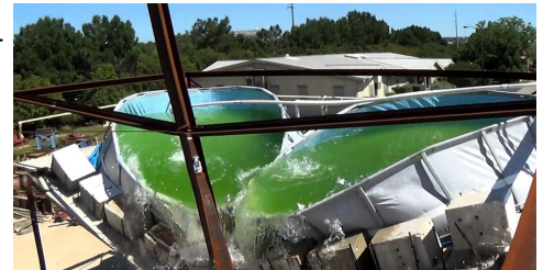
The floor slab at the moment of collapse
