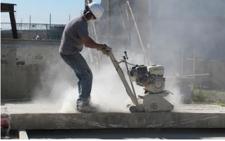
The physical autopsy was conducted using a Scarifier (aka the loud dust-maker)
