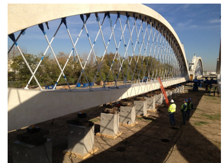
Upward jacking on one of the arches
