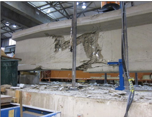
Failure of control specimen
