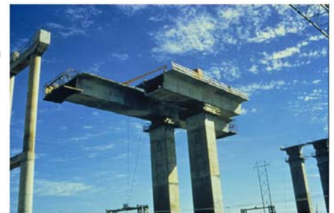
Bridge under construction in Corpus Christi
