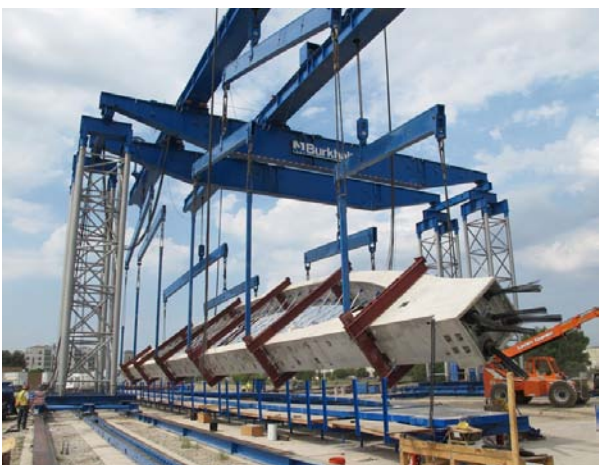
First arch being rotated
