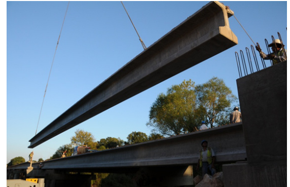
Instrumented girders being installed at TxDOT bridge construction site
