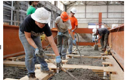
Casting the 12 (non-prestressed) slabs in the prestressing bed
