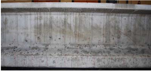
Service load testing of a 0-6374 specimen
