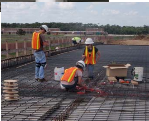
Mounting solar panel on side of bent cap (above) and installing gages on the deck (right)
