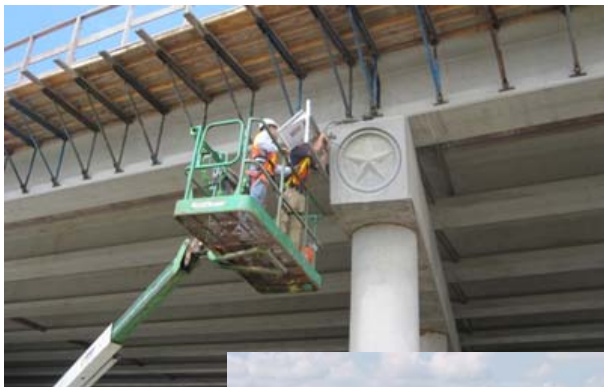
Mounting solar panel on side of bent cap (above) and installing gages on the deck (right)
