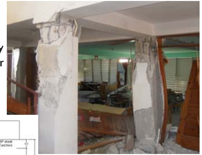
RC columns damaged by Haiti earthquake in 2010 (right) and scheme of the retrofit for one RC column (bottom)
