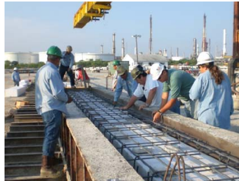
Pros at Precast Yard
