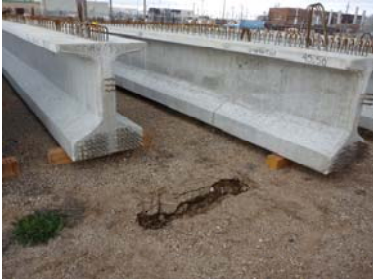
Lubbock pavements are not designed for 19 kip point loads, FYI
