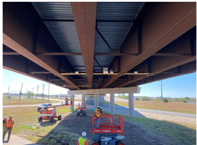
Live Load Testing on the Chisholm Trail Parkway Bridge
