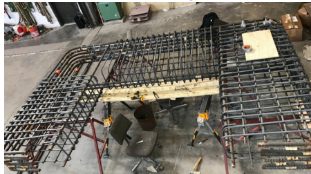
Curved-bar-node Steel rebar cage
