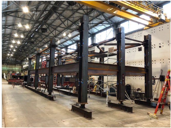
Test Setup during erection
