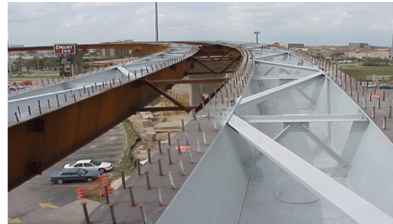
Shear studs on tub girder flange
