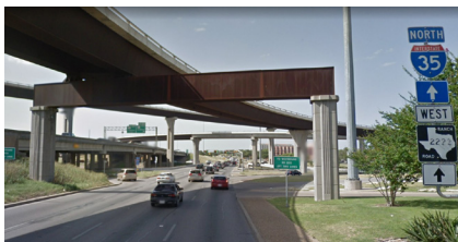
Steel box straddle cap over north I-35 frontage road (Google Maps)
